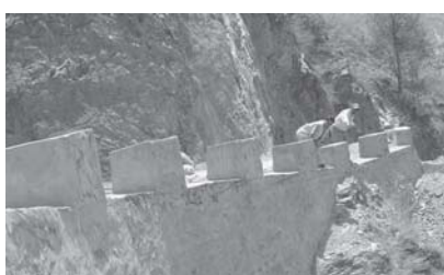
Masonry wall in Bagbazar-Bagarkot road, Darchula
